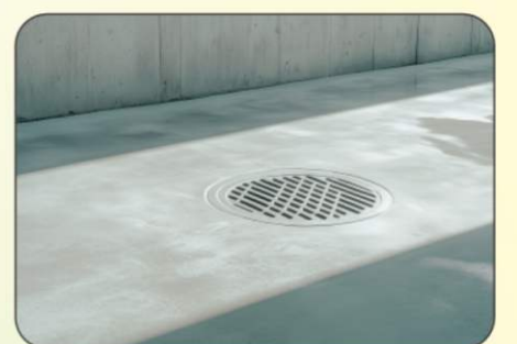
CC Road with CC Drain
